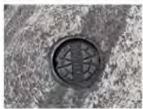
Q-25 Survey 9" cover in front of 7671 Diamond Pointe Way.
