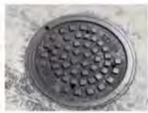
Q-26 Sewer 27" cover in front of 7671 Diamond Pointe Way.
