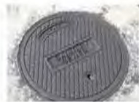
G-12 Sewer cover plate 27" in front of 7555 South Claridge Pointe Parkway.
