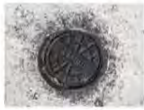
N-22 Survey 9" cover in front of 150 Platinum Pointe Way.
