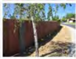
5.12 North of 181 Platinum Pointe Way facing Lancaster Drive.
