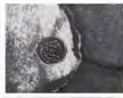
G-8 Water 9" cover in front of 3 Brookshire Drive.
