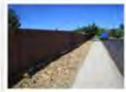
5.6 North of 121 Platinum Pointe Way facing Lancaster Drive.
