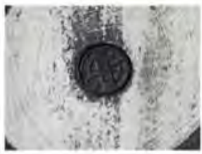
H-13 Survey 9" cover plate in front of 7601 South Claridge Pointe Parkway.
