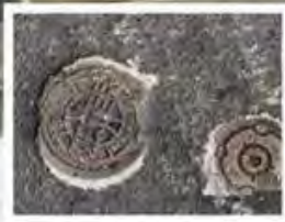
A-1&2 VALVCO 6 1/2" cover and 9" Water cover at entrance to North Claridge Pointe Parkway.
