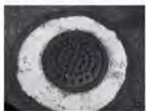
T-29 Sewer 27" cover in front of 7610 Diamond Pointe Way.
