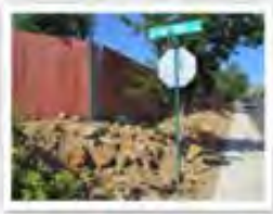
4.1 North corner of 7660 South Claridge Pointe Parkway facing Lancaster Drive.
