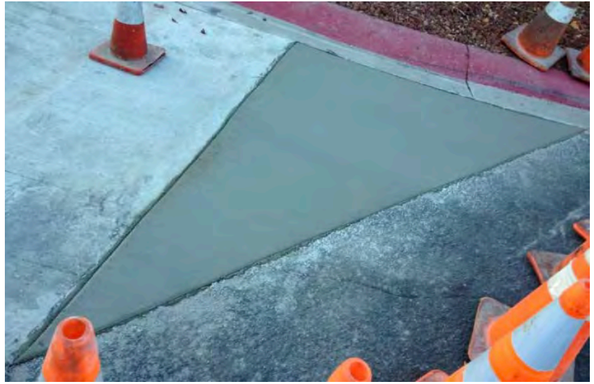
Gutter repair and swale extension at 7500 Diamond Pointe Way installed November 2014
