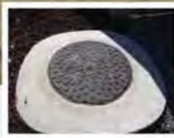
C-4 Sewer cover plate 40" diameter located off road at south west corner of 7740 NCP.
