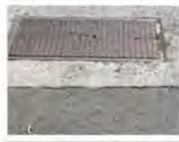
J-15 Access cover plate in North Virginia Street presumably for North Claridge Pointe.
