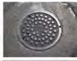
F-7 Storm drain 27" cover at intersection of Brookshire and North Claridge Pointe Pkwy.
