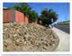
3.1 East of 7500 South Claridge Pointe Parkway facing North Virginia Street.
