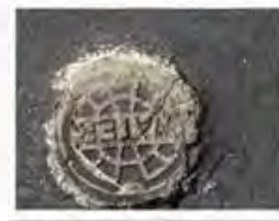
I-13 VALVCO 6 1/2" cover outside of fire gate at entrance to Brookshire Drive.
