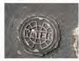
I-14 Water 9" cover outside of fire gate at entrance to Brookshire Drive.
