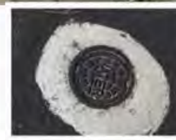
D-5 Water 9" cover in front of 7805 North Claridge Pointe Parkway.
