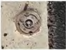
C-5 VALVCO 6 1/2" cover plate next to driveway at 7500 Diamond Pointe Way.
