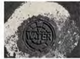
C-8 Survey 9" cover plate next to driveway at 7500 Diamond Pointe Way.
