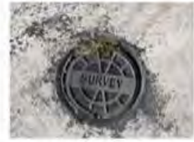
B-4 Survey 9" diameter near 7500 Diamond Pointe Way.
