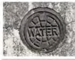
G-11 Water 9" cover in front of 3 Brookshire Drive.
