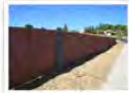
5.10 North of 161 Platinum Pointe Way facing Lancaster Drive.
