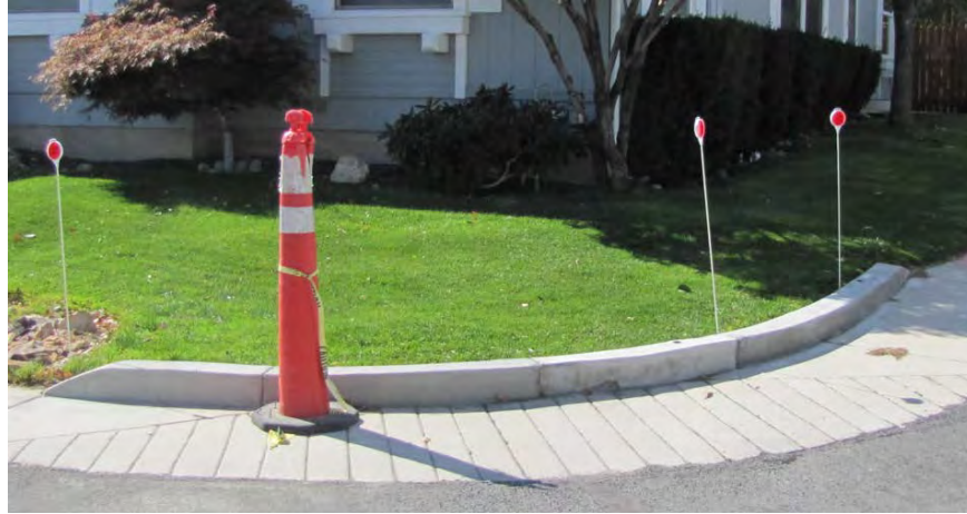
7895 North Claridge Pointe Parkway Installed July 2013 and Repaired October 2016
