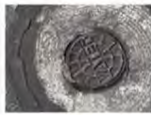
O-23 - Water 9" cover in front of 161 Platinum Pointe Way.
