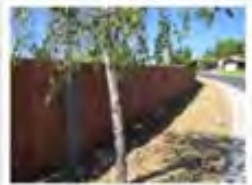
5.12 North of 181 Platinum Pointe Way facing Lancaster Drive.
