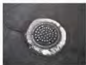
V-31 Sewer 27" cover in front of 7541 Diamond Pointe Way.
