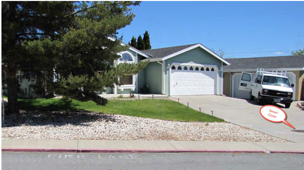
Association Owned Property for Future Parking Area
