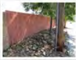
6.2 South of 7705 North Claridge Pointe Parkway facing Lancaster Drive.
