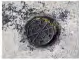
B-3 Survey 9" diameter near 7500 Diamond Pointe Way.
