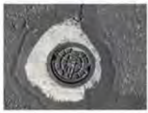
J-17 Water 9" cover in front of 7690 South Claridge Pointe Parkway.
