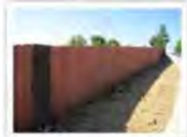
5.14 North of 191 Platinum Pointe Way facing Lancaster Drive.
