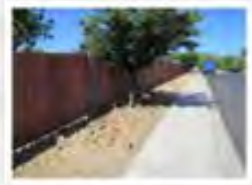
5.5 North of 111 Platinum Pointe Way facing Lancaster Drive.
