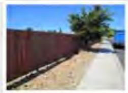
5.7 North of 131 Platinum Pointe Way facing Lancaster Drive.
