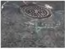
A-1 Sewer cover plate at Wellington Way. This is the tie in from South Claridge.
