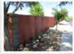
5.4 North of 101 Platinum Pointe Way facing Lancaster Drive.
