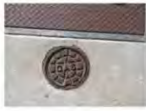
I-14 Gas 9" cover in driveway of 7670 South Claridge Pointe Parkway.
