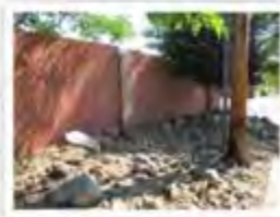
6.3 South of 7705 North Claridge Pointe Parkway facing Lancaster Drive.
