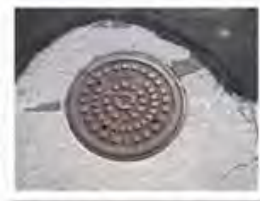
E-6 Sewer 27" cover in front of mailboxes in North Claridge Pointe.
