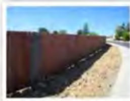
5.13 North of 181 Platinum Pointe Way facing Lancaster Drive.
