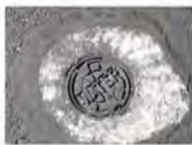
F-11 Water 9" cover plate in front of 7550 South Claridge Pointe Parkway.
