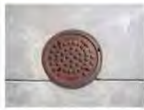
I-15 Sewer 27" cover in driveway of 7670 South Claridge Pointe Parkway.
