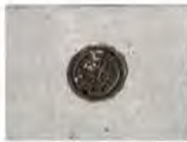
E-10 Gas 9" cover plate in the driveway of 7535 South Claridge Pointe Parkway.
