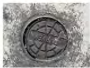
U-30 Survey 9" cover in front of 7590 Diamond Pointe Way.
