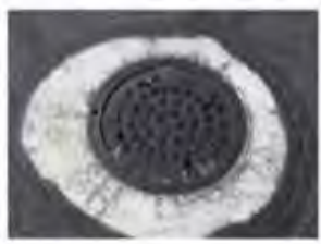
M-21 Sewer 27" cover in front of 121 Platinum Pointe Way.
