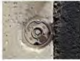
C-6 VALVCO 6 1/2" cover plate next to driveway at 7500 Diamond Pointe Way.
