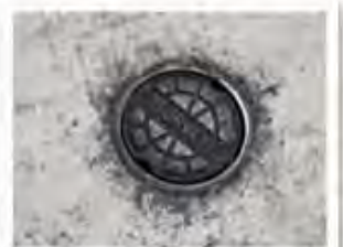
W-32 Survey 9" cover in front of 7520 Diamond Pointe Way.
