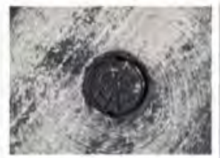
P-24 Survey 9" cover in front of 181 Platinum Pointe Way.
