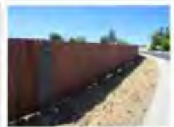
5.13 North of 181 Platinum Pointe Way facing Lancaster Drive.
