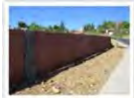
5.11 North of 171 Platinum Pointe Way facing Lancaster Drive.
