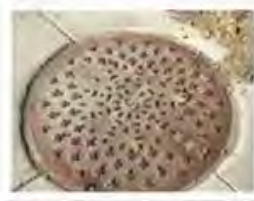
K-16 Sewer cover plate 40" diameter located in sidewalk next to N. Virginia and behind 7740 NCP.
