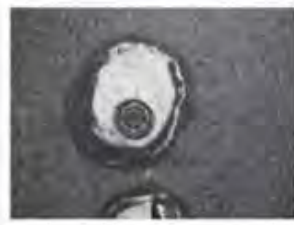
L-19 - Survey 9" cover in front of 101 Platinum Pointe Way.
