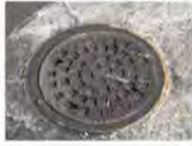
A-2 Sewer cover plate 27" diameter located outside of the fire gate facing Wellington Way.
