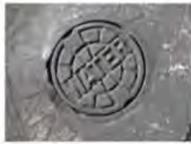
C-7 Water 9" cover plate next to driveway at 7500 Diamond Pointe Way.
