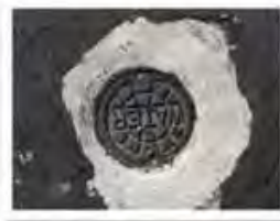
H-12 Water 9" cover in front of 1 Brookshire Drive.
