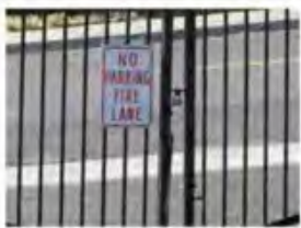
B-5 No Parking Fire Lane Sign on fire gate at Wellington & SCP facing south.
