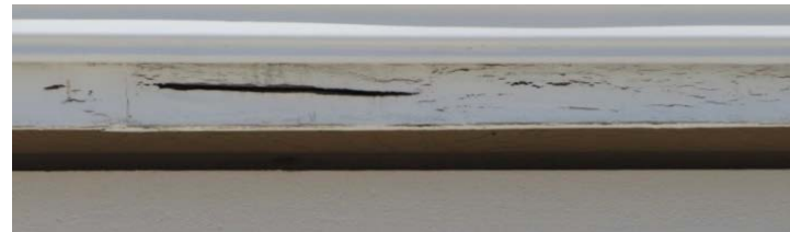
Examples of blistered paint and bare spots.
