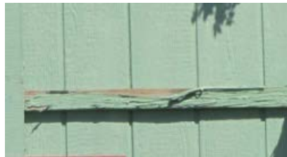
Examples of blistered paint and bare spots.
